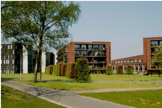
New apartment buildings integrated in the park
